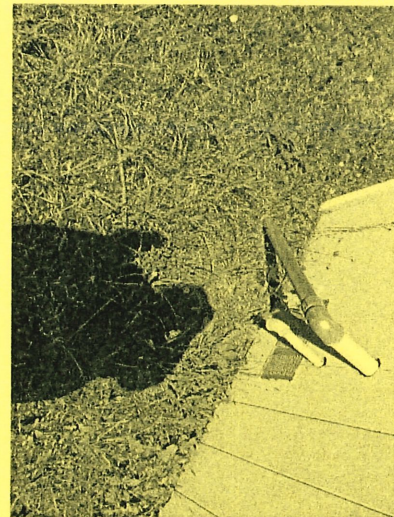
Drain outlet for PRV - needs screen
