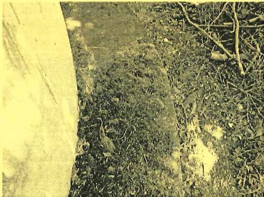
Moss on foundation of Tank 1
