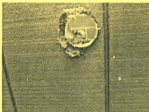
Opening in Well 2 enclosure
