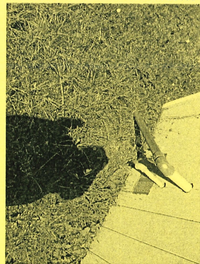
Drain outlet for PRV - needs screen
