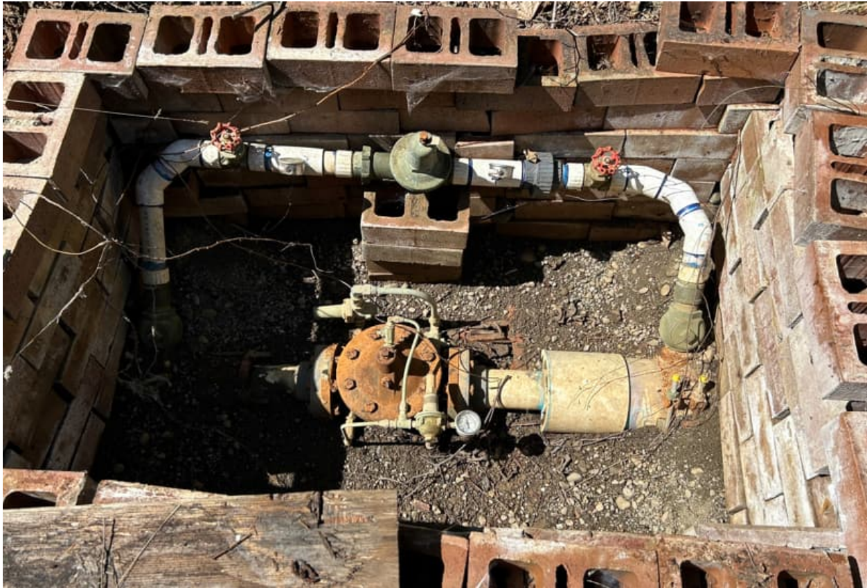
Figure 3-2 Existing PRV Station
