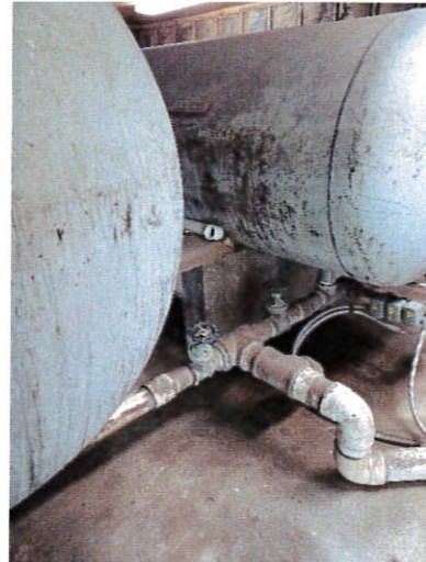
Hydropneumatic Tanks
