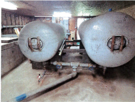
Back of hydropneumatic tanks
