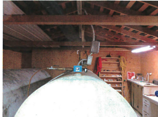
Air compressor input and float switch controls for hydropneumatic tanks.
