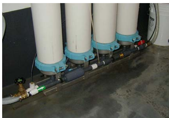
The picture on the left shows one set of filters. Source water enters through the hose inlet in the wall, passes through a flow meter, past a chlorine injection point, through an in-line static mixer, into the inlet manifold, down through the filter media. Product water is discharged through the wall. The pail holding the sodium hypochlorite solution can be seen to the right of the filter vessels and the in-line chlorine analyzer is on the wall above the NaOCl container. The sample ports and analytical equipment is forward of the chlorine analyzer. A second container of Ferric Chloride solution and feed pump is provided for pilot testing for arsenic removal.
