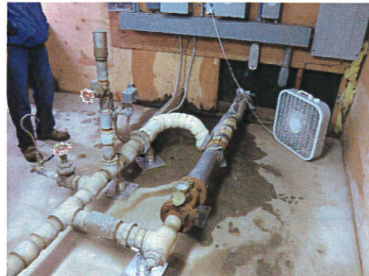
Temporary plumbing from a break the previous weekend.
